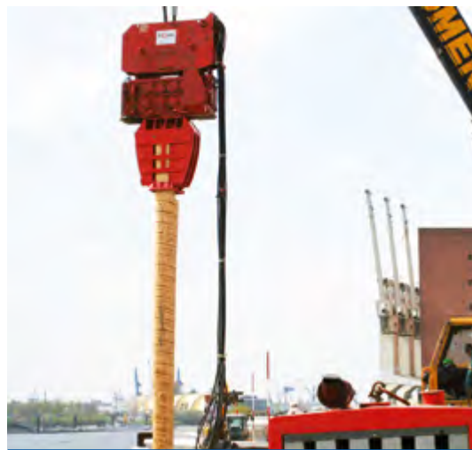
30HFV Vibrodriver driving wooden piles at the entrance of the Marina, Hamburg-Germany.
